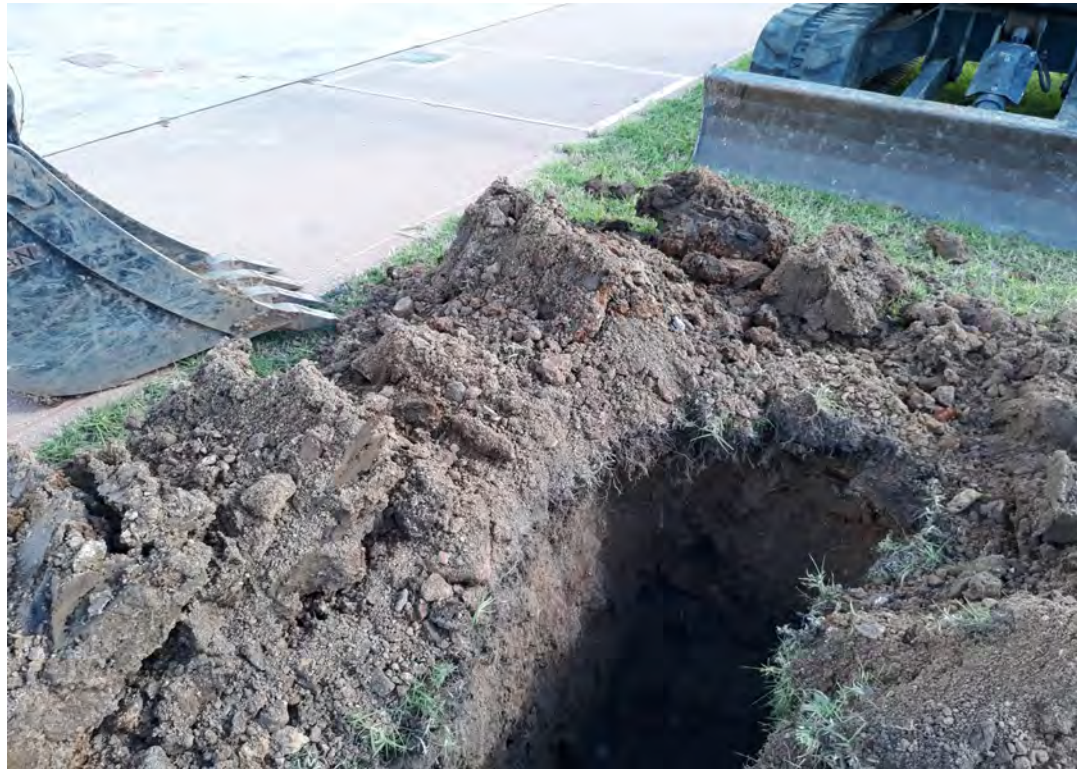
Photo 3: View of pit 505
